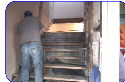
Leicester Jones and Greg Swain removing the old stairs
