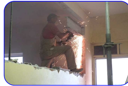
Cutting through a steel beam
