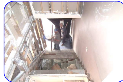
Leicester Jones and Greg Swain removing the old stairs
