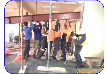
Installing a large steel beam
