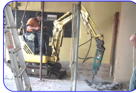
Jordan uses a jack-hammer
